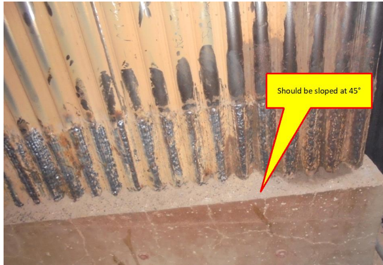
Photo 49: Photo shows the repair of weld overlay zone in wing wall SH. The mistake here is that the refractory should be sloped at 45° to allow free flow of solids without much resistance.
