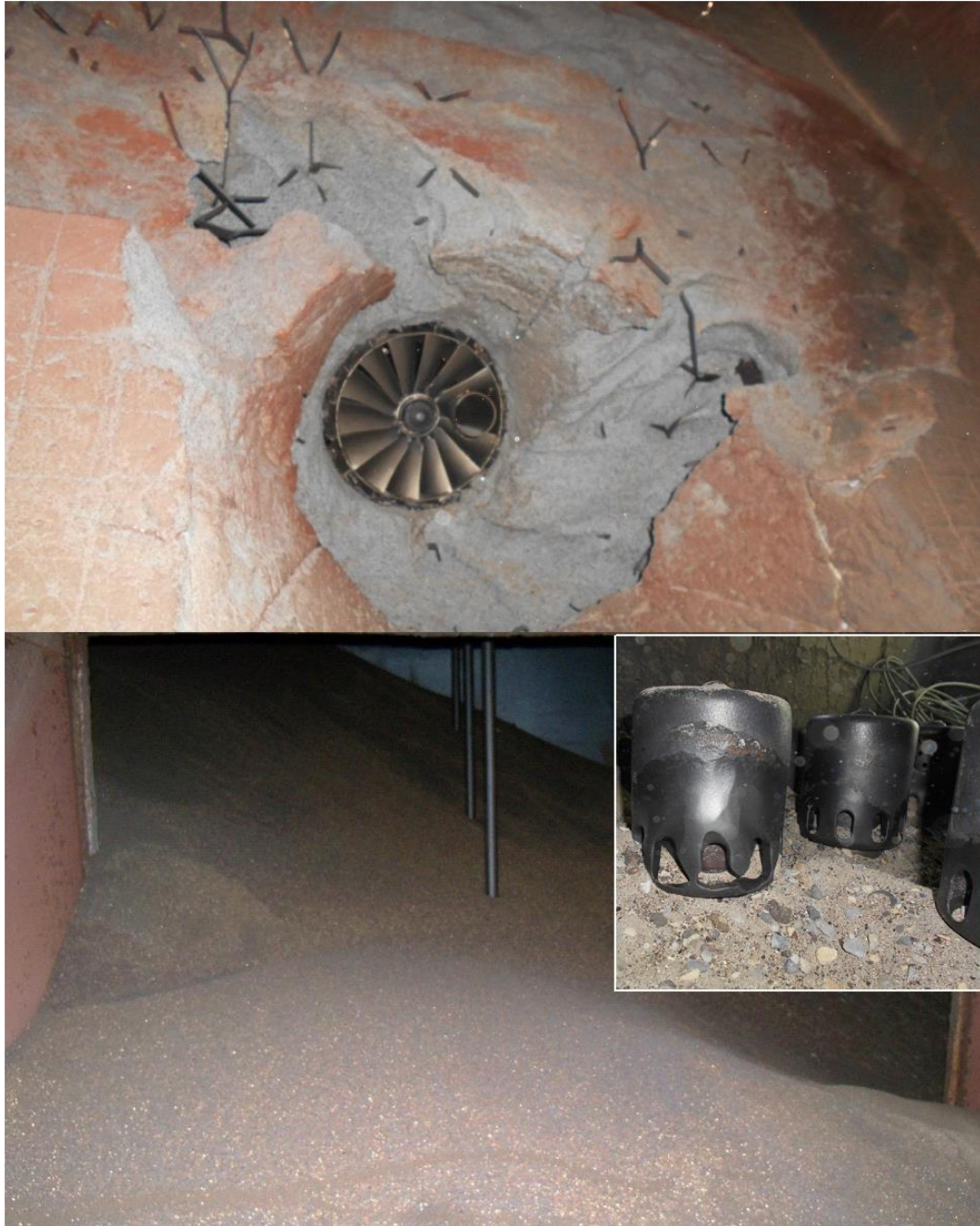
Photo 12-14: Thick refractory in CFBC furnace walls is prone for spalling because thermal expansion. The air nozzles get eroded when the spalled refractory fall in between the nozzles and obstruct the air path as they get stuck near / at air nozzle openings. Air nozzle failures cause combustible bed material seepage in to the windbox. This is a serious hazard starting from simple refractory defects. Bottom photo shows the accumulation of bed material inside the windbox.
