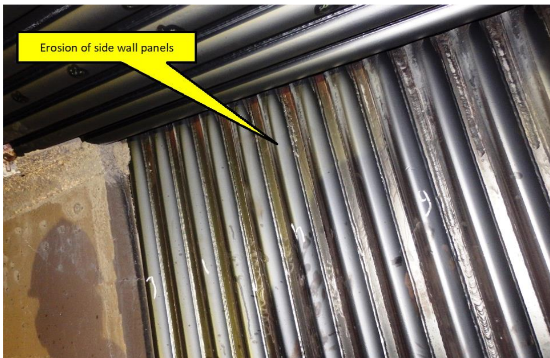
Photo 6: The above photo shows the erosion of side wall panels in the boiler with cyclone entry configuration as in figure 3.
