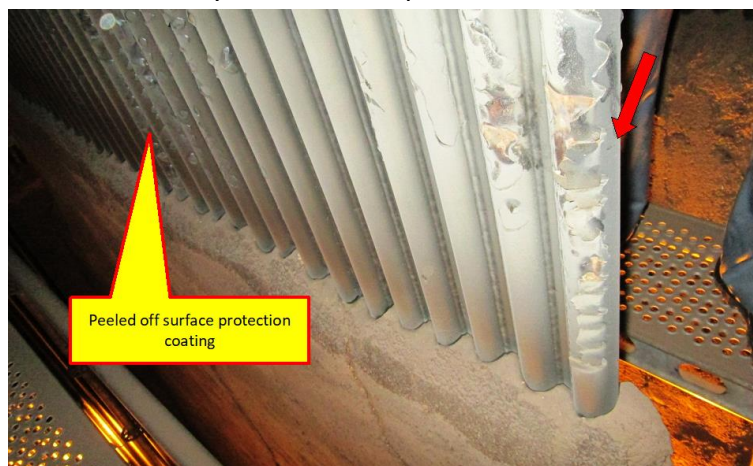
Photo 48: Photo shows the peeling of the HVOF spray over the wingwall evaporator panel. Field repair is not successful, unless it is executed with complete removal of previous coating.
