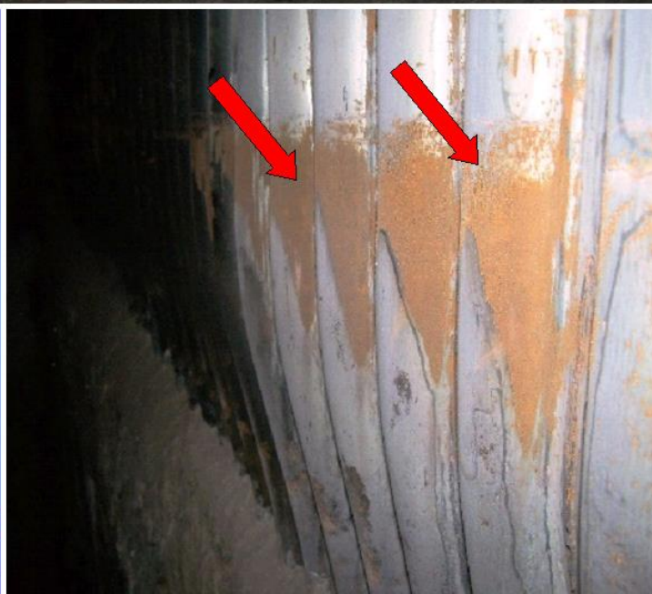
Photo 30 & 31; Figure 20: The top photo shows the erosion of tubes when a panel is inclined / out of verticality. Bottom photo shows the case of out of verticality of bottom panel at the field joint. In the figure the erosion mechanism is illustrated.
