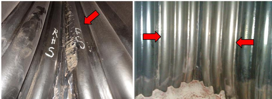
Photo 15 & 16: Both the photos above show erosion of corner tubes in CFBC boiler. The location depends on the load factor and the cyclone outlet configuration. In addition, the corners of CFBC boilers generally have defects on fin closures. By applying the corner refractory, the corner tubes can be protected. See figure 9 below.
