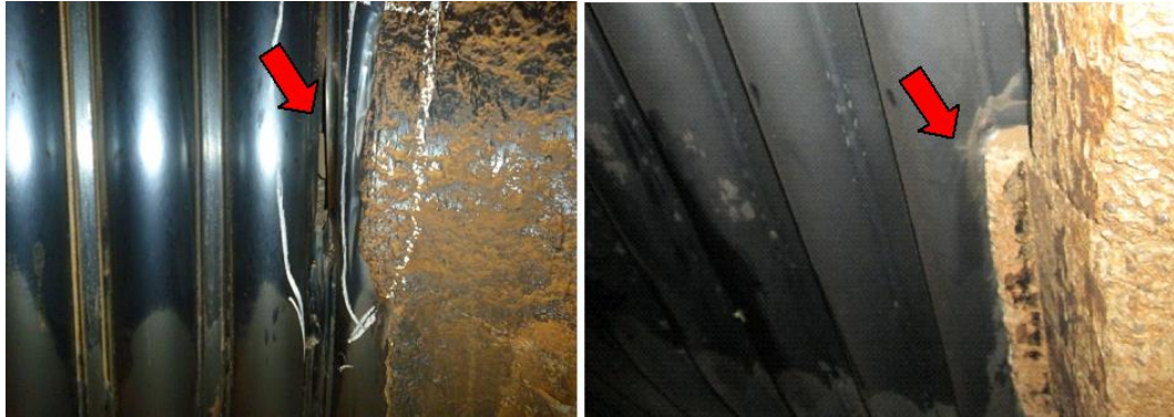
Photo 17 & 18: While the CFBC boiler demands a corner refractory detail for protection from erosion, improper design, improper application cause localized erosion. Localized deep cuts are seen in places of improper refractory tipping. Metal filling is to be done to stop the growth of the cut.
