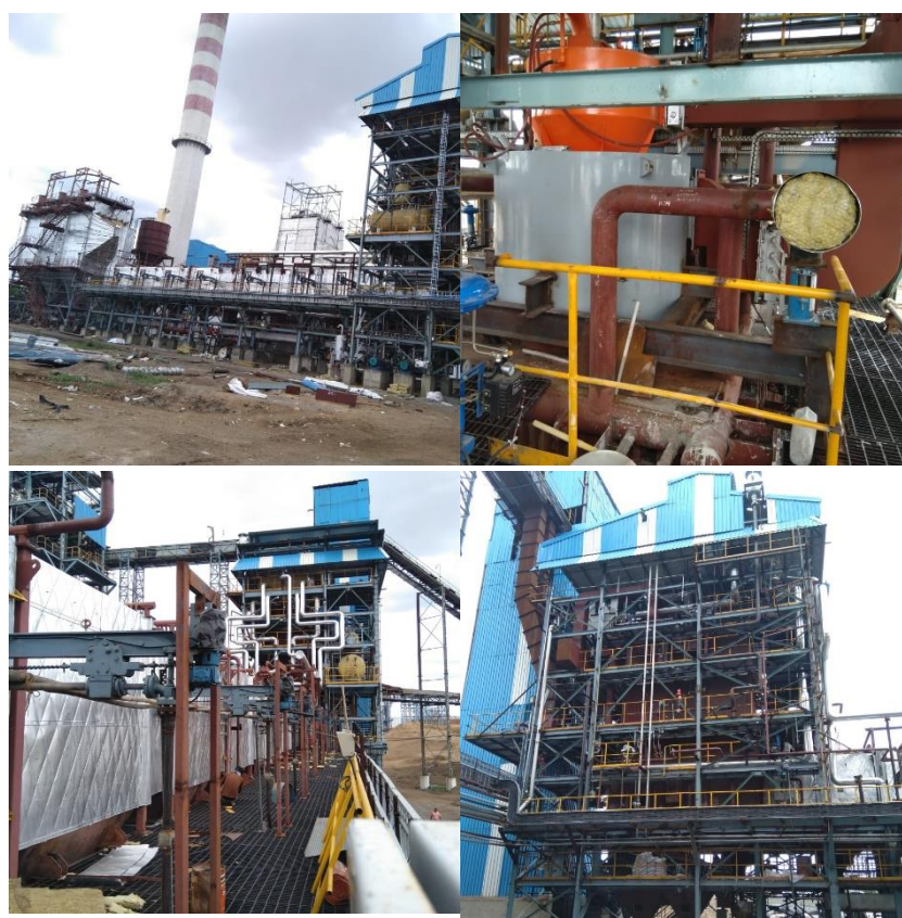
15tph, 45 Kg/Cm 2 g, 410°C Bio-Methanated Spent Wash Incineration Boiler at Utopian Sugars Ltd., Solapur (*PATENTED)
