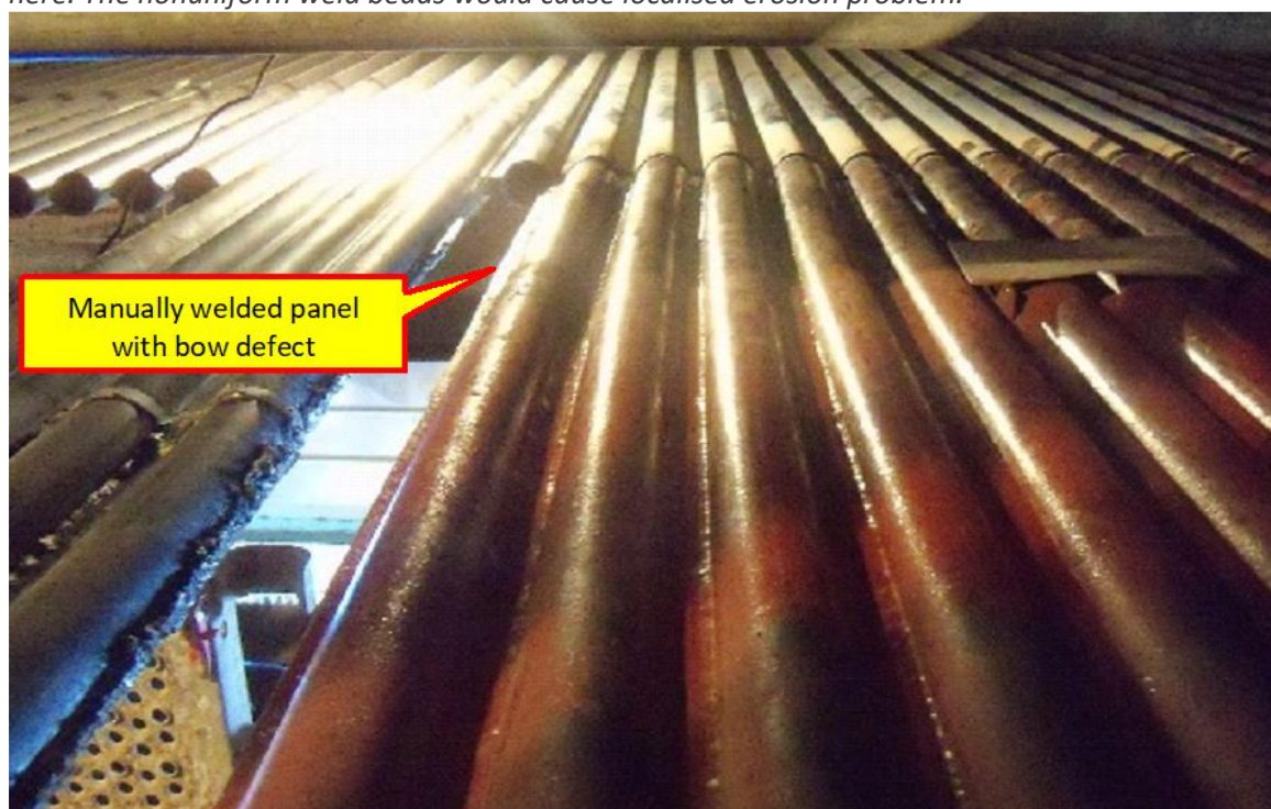
Photo 35: Photo shows the out of alignment of manually welded panel below the original machine welded panels. Boilers owners have to procure the spare panels only from parties who would deliver the panels duly welded in mechanized welding machine. Panel replacement team should be clear about the quality requirements at field.
