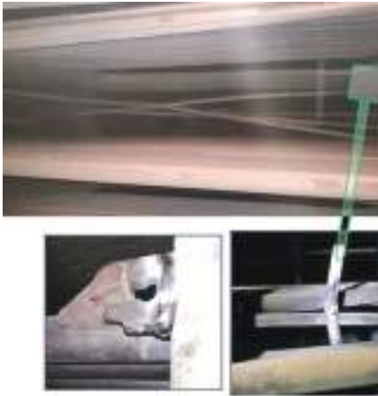
Figure 11: Platen zone spacer failure
