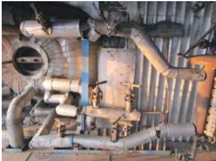
Figure 10: Drain line connections
