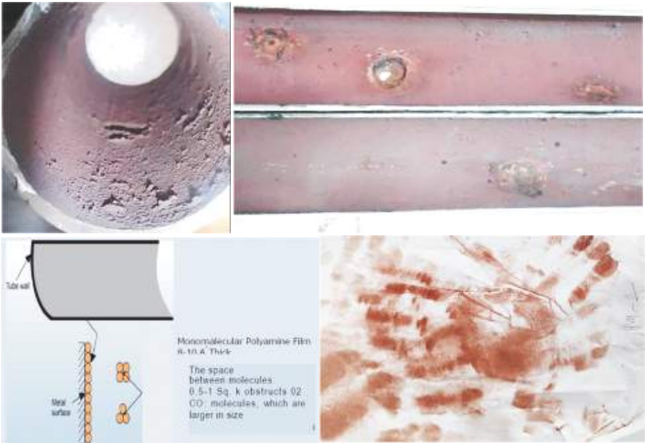
Photo 12 -15: Paper mill boiler suffered from under deposit corrosion after prolonged operation without appropriate descaling of the boiler. The iron oxides get transported from machine cylinders. Use of filming amine generally reduces the boiler corrosion rate. The rub off is from inside of the drying cylinders.
